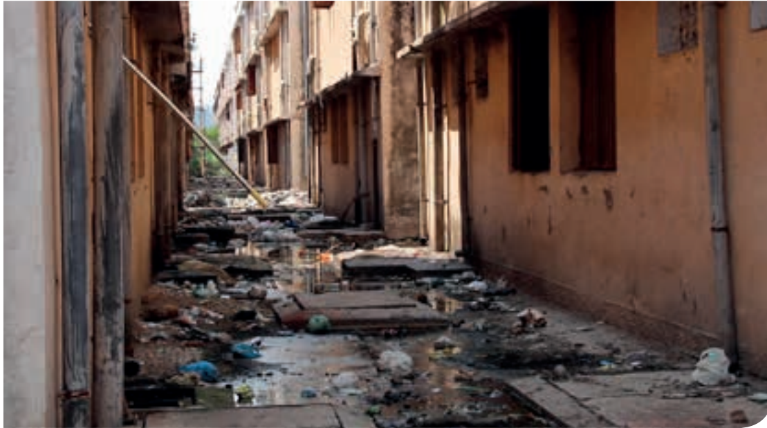
People living in informal settlements in India are relocated to inappropriate housing far from their communities.
